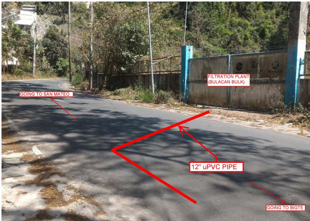
Location of the Proposed Tapping point from the bulk supplier and starting point of the 300mm diameter transmission/distribution pipeline
